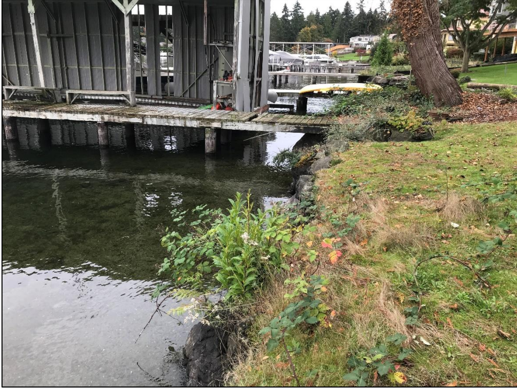
Photo 3. View of shoreline and bulkhead from northwest property line looking southeast.
