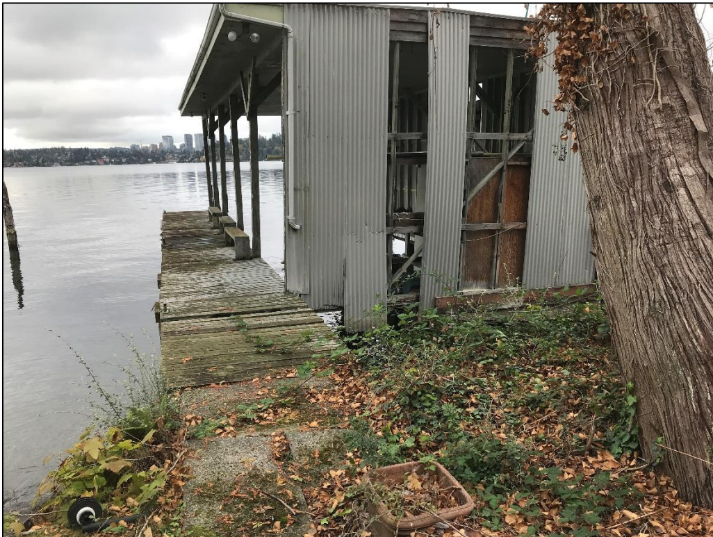
Photo 2. View of pier and moorage cover from pier entrance looking northeast.
