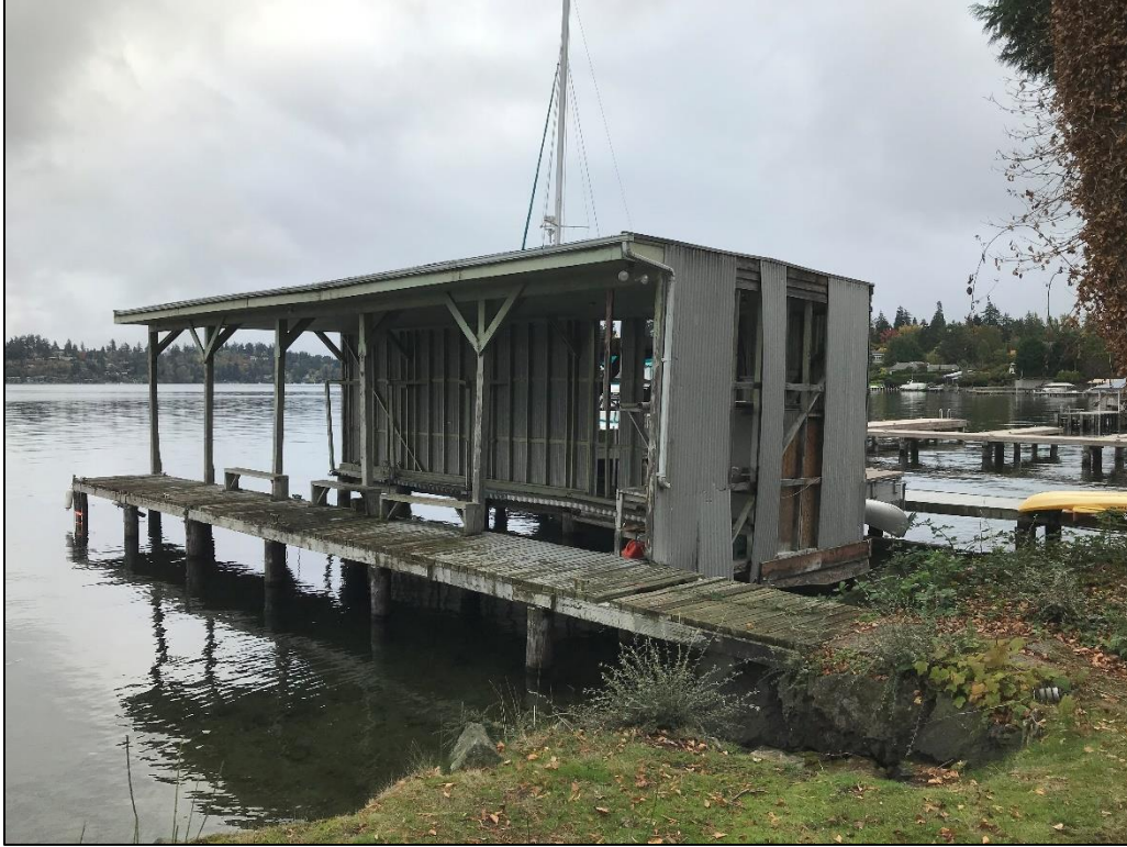
Photo 1. View of pier and moorage cover from shoreline looking east.
